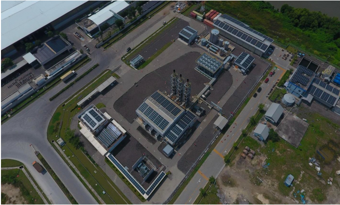
Exhibit 01. ESG Initiatives: KEK-JIPE installs 764 solar panels
