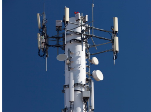
Pole/monopole: Composed of Easy Macro (<10m), Micro Pole (MCP) (12-20m) and Mini Macro (21-30m)
