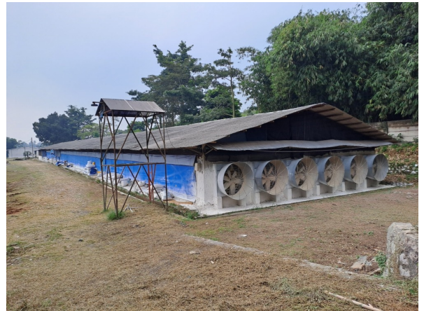
Exhibit 04. Large fan installations on the closed house system
