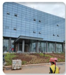
OPPO Office & Factory
